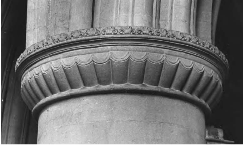
Plate 32 Capital and abacus of a pier in Malmesbury Abbey, Wiltshire. The repetitive palmette motif, almost identical to similar designs found in Ancient Egyptian and Greek work, decorates the abacus. This pier was associated with a statue of the Virgin Mary and dates from c. 1170. Photograph of 1981 (JSC).
